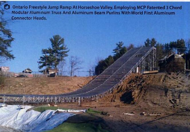
Ontario Freestyle Jump Ramp At Horseshoe Valley, Employing MCP Patented 3 Chord Modular Aluminum Truss And Aluminum Beam Purlins With World First Aluminum Connector Heads.
