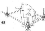
2. With a level begin by levelling one transom, then go diagonally to the ledger on adjoining base collar. Then level the ledger and continue around base. Measure the horizontal distance between slots on top of mouthpieces in both directions. Adjust for square. Drive home all wedges. Use of a plan brace eliminates measuring. No further leveling or plumbing of the scaffold will be required.
